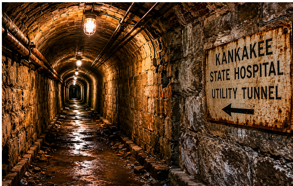
Tunnels beneath the Shapiro Developmental Center
